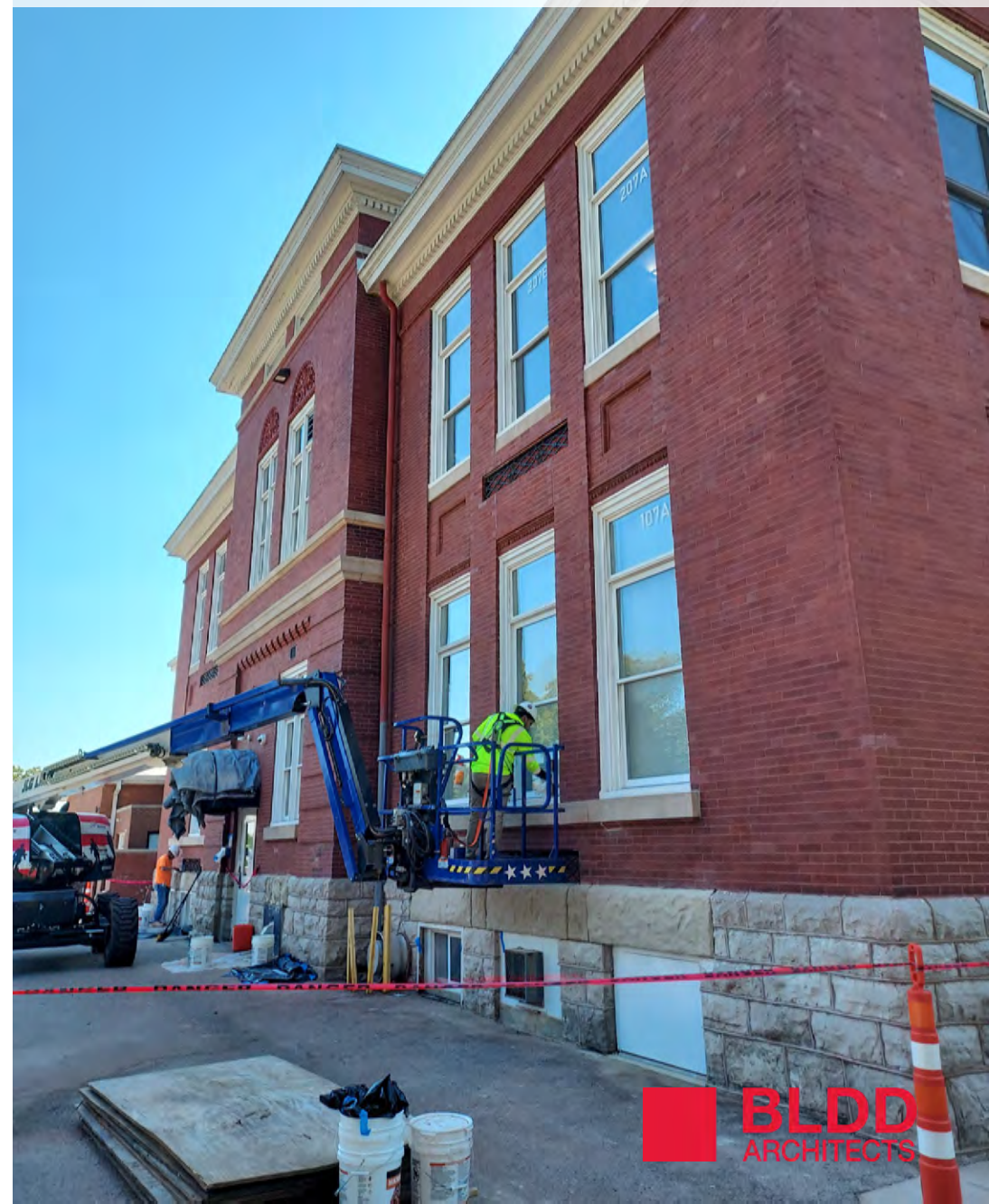
Administrative Center | St. Charles, MO
